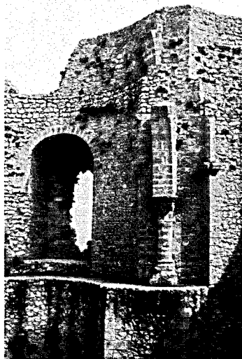
Etampes (Essonne). Guinette Tower, built in the 12th century, was decorated in the 13th with rare elegance. Here a corner of the great hall (upper story) is shown, well lighted and equipped with a series of arches that made it possible to dispense with the central pillar.
